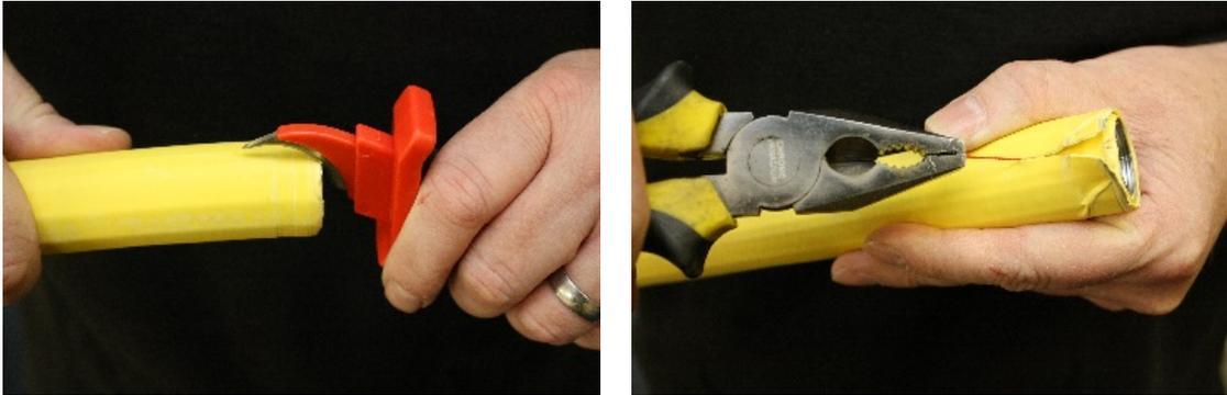
**SCORE AROUND CIRCUMFERENCE OF PIPE:** Use a utility or cable knife to lightly score around the circumference of the pipe. **DO NOT FULLY PENETRATE THE OUTER COVER WITH THE KNIFE BLADE**
